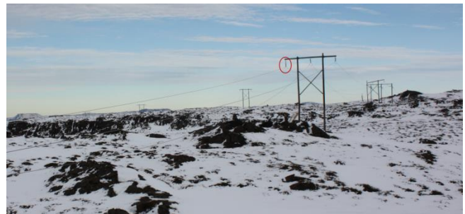
Fig. 8. Suspension tower in 132 kV KS1 with measuring equipment in left phase at Reykjaheiði site.
