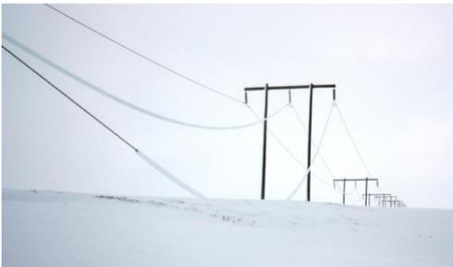
Fig. 1 Wet snow icing on power line in winter 2012.
