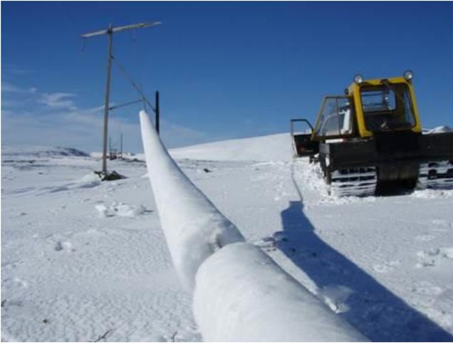
Fig. 8 Site No. 1 (Kop100). Failure of power line during wet snow icing in 2012, case 3-a).
